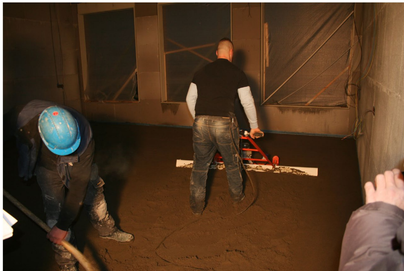
Figure 2. The manually moved electrical screed levelling machine.
