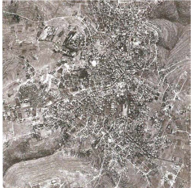
Figure 10: Ramallah as a Town, 1967, Source: Atlas of the Conflict
