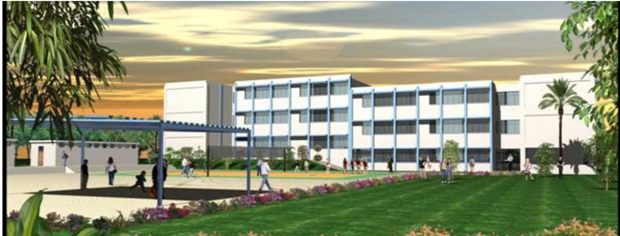
Figure 16: Double-Sided Hammerhead School, Source: UNRWA office Amman
