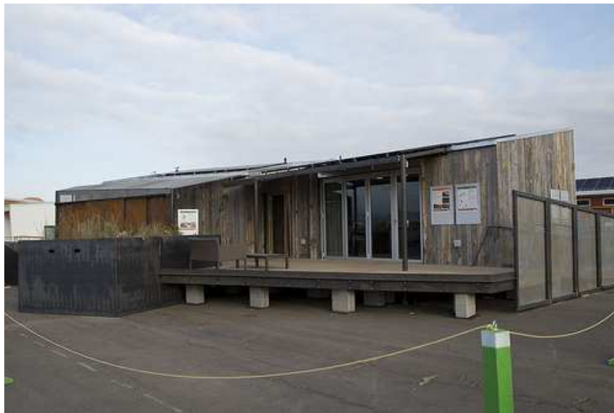
Figure 2. South Face of DesertSol
