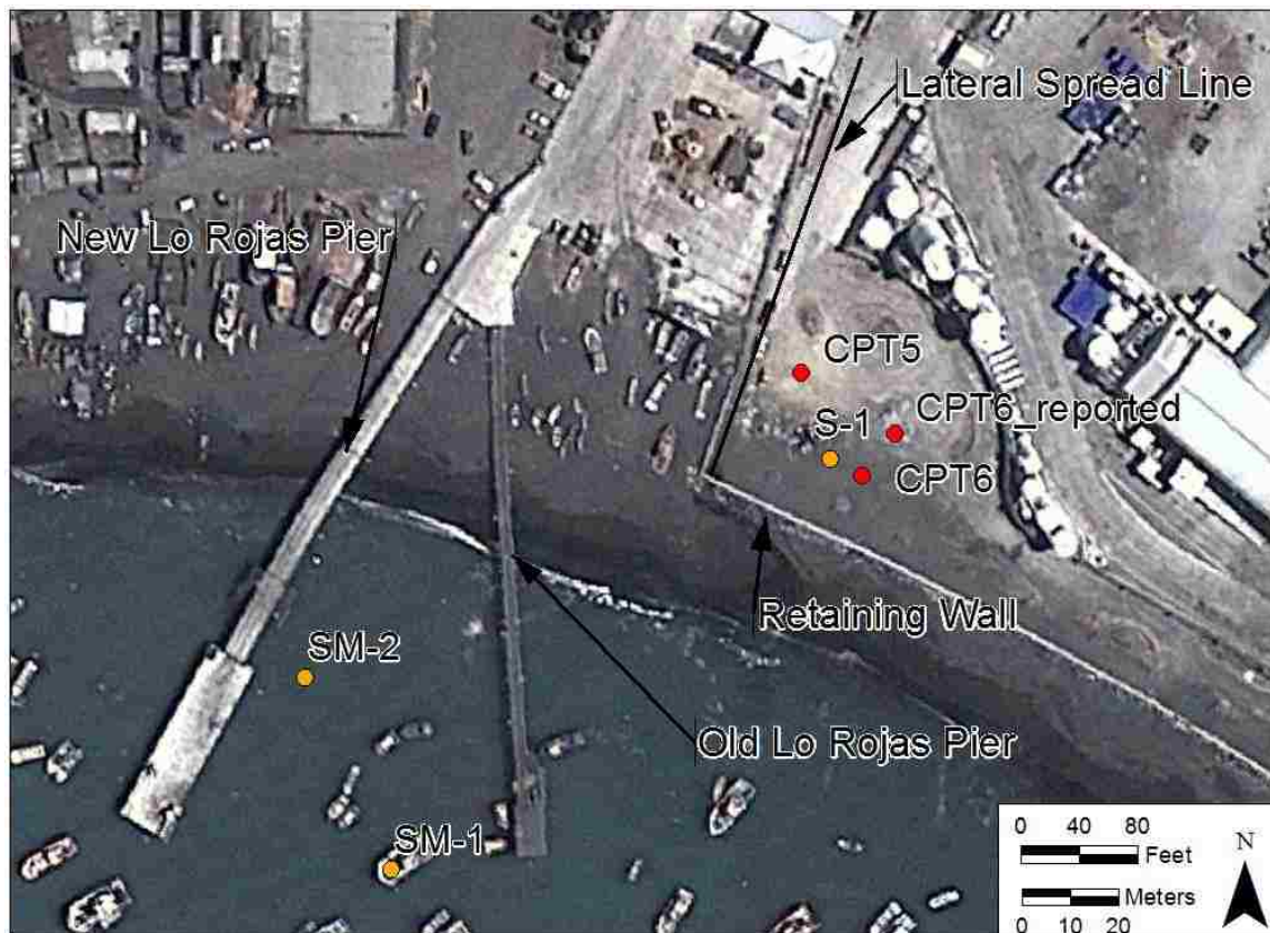
Figure 18. Lateral spread line, SPT and CPT locations near Lo Rojas pier and lateral spread line.
